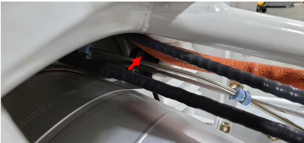
Figure 3.2.3 – RH Upper Engine Isolator
